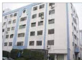
MEAN WELL GUANGZHOU TIANHE R&D CENTER
